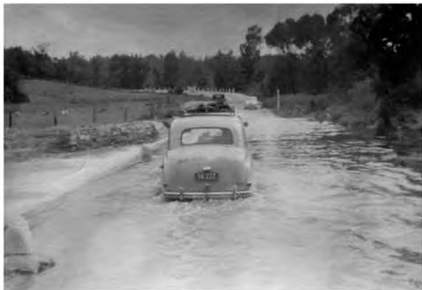
River in flood, water above the bridge
